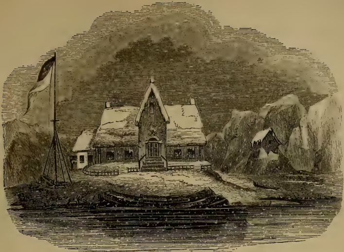
INSPECTORS' HOUSE, LIEVELY.
